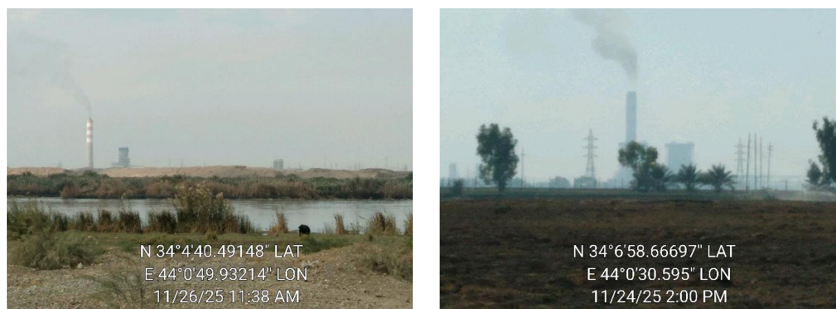
Figure 4-13: Photographs of Samarra Diesel Power Plant
