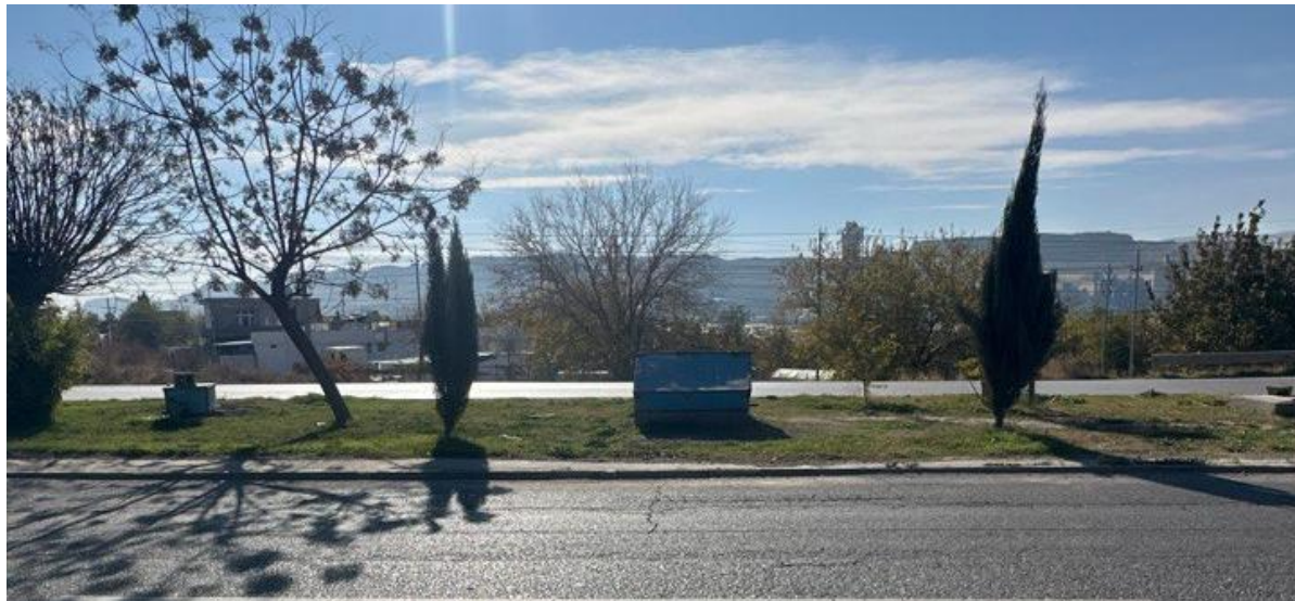
Figure 4-41: Groundwater well in the median
